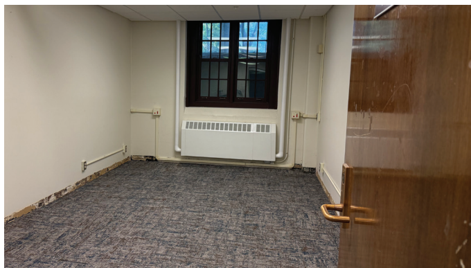
New carpet was installed in faculty offices. New doors with uniform nameplates will be added by winter break.
