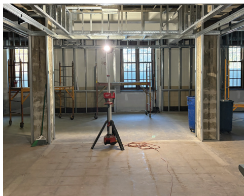
Renovations included knocking down walls to combine Rooms 1, 2, and 3. Substantial completion is scheduled for mid-December.
