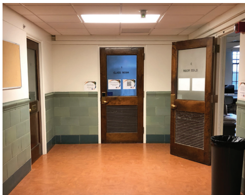
Rooms 1, 2, and 3 on the east wing were two smaller classrooms and a faculty office.
