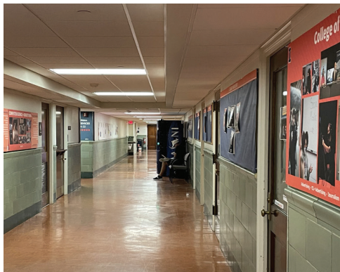
Gregory Hall lower-level corridor before renovations.
