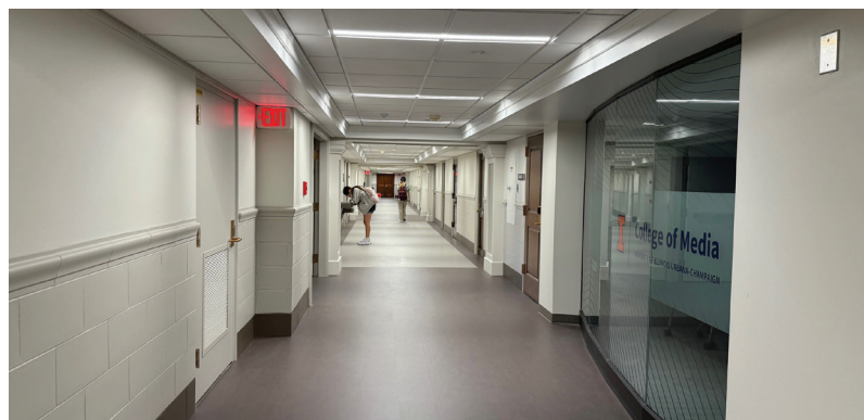
Corridor renovations were completed before the first day of classes. New digital signage will be installed this spring.
