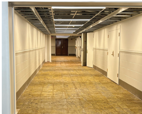
Lights installed and floor removed.
