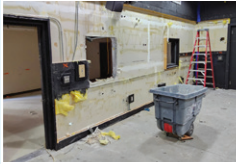
Studio wall being removed to reconfigure into one large window between the studio and newsroom.
